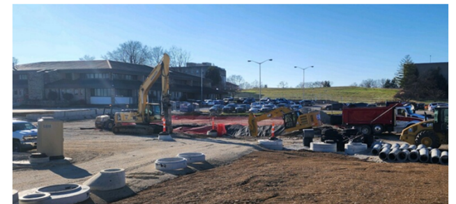
Hopewell East Construction Photo
