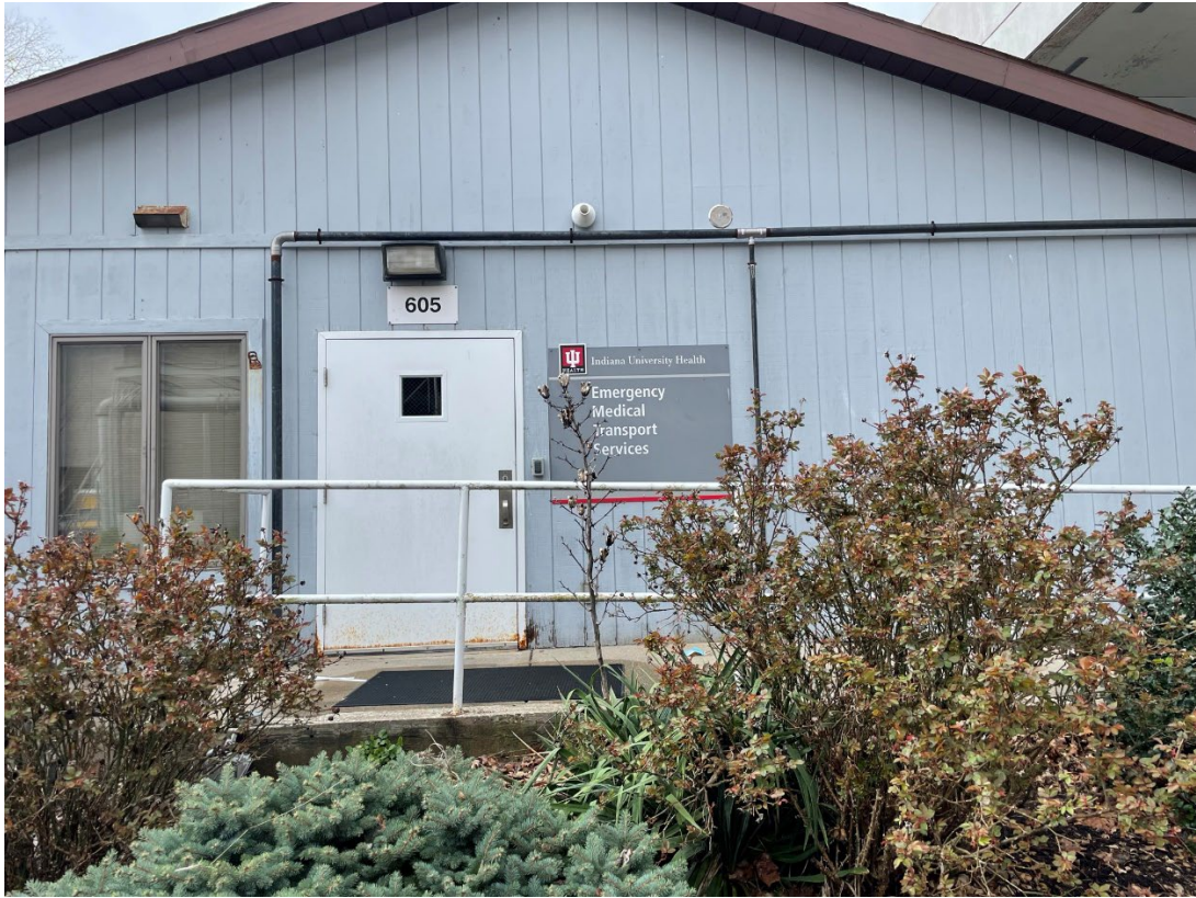
Photo 3: Subject Site – 605 W. 1 st Street, EMT Services
