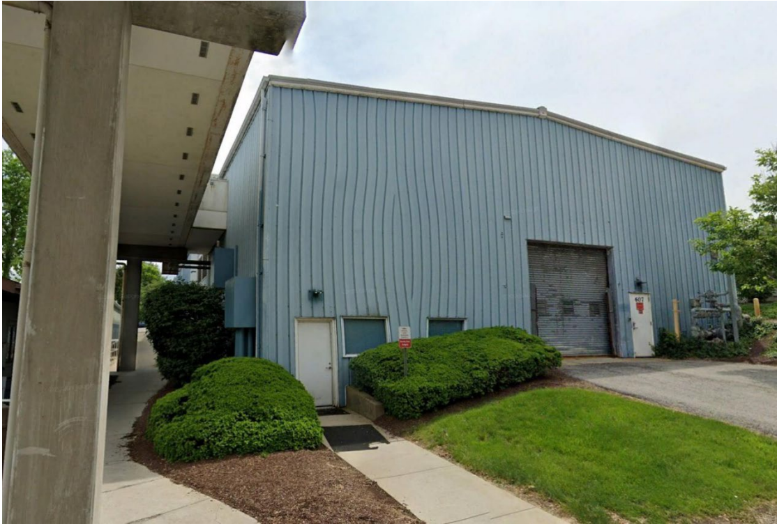
Photo 1: Subject Site – 607 W. 1 st Street, Power Generation Facility.
