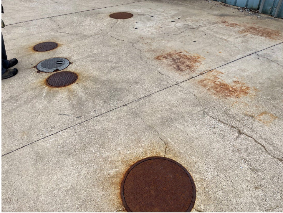
Photo 5: Subject Site – Fill ports west of power generation facility.
