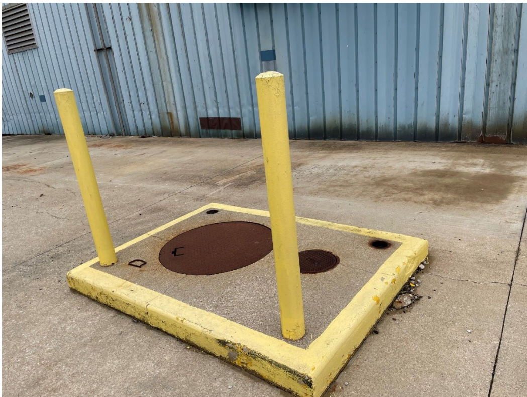
Photo 12: Subject Site – Possible wastewater system west of power generation facility.
