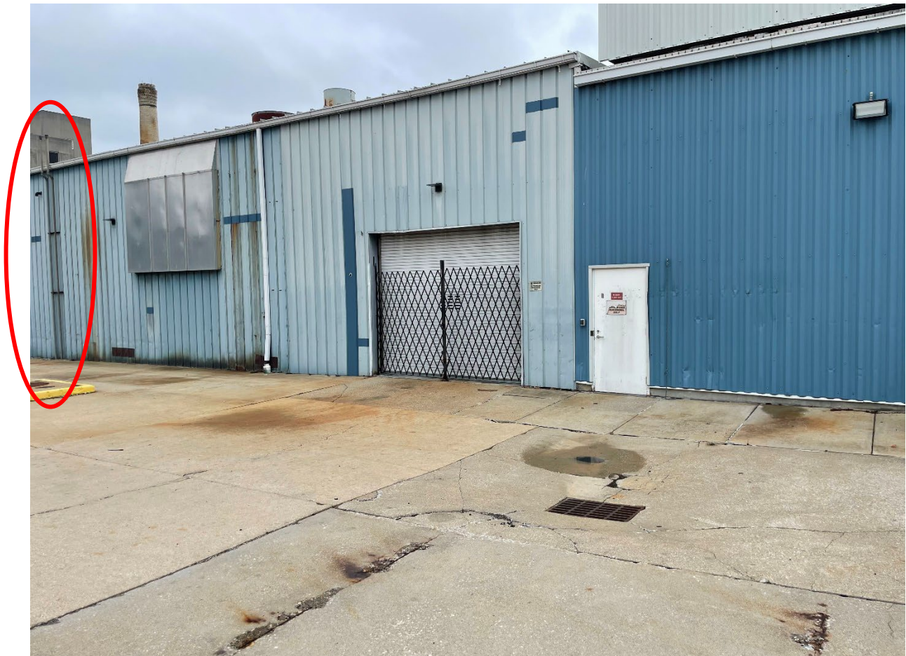
Photo 6: Subject Site – Vent pipes west of power generation facility.
