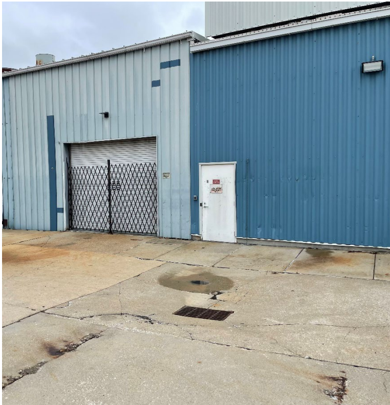
Photo 11: Subject Site – Storm water drain west of power generation facility.
