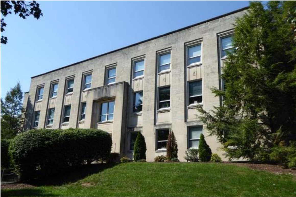
Photo 1 The main elevation faces east.
