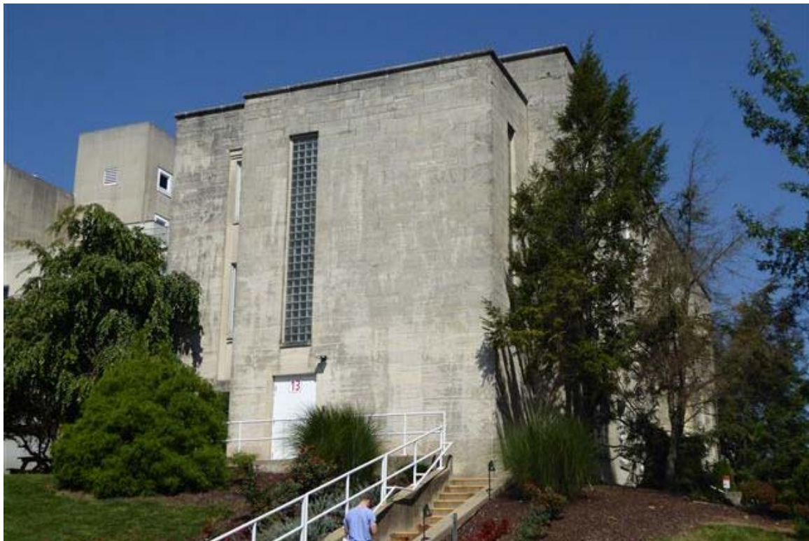
Photo 2 A stairwell extends off the south elevation.
