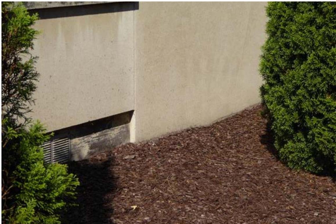
Photo 48 ...typically extend well up onto the face of the limestone.
