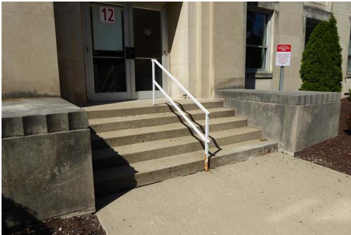
Photo 40 As are the steps into the main entrance.
